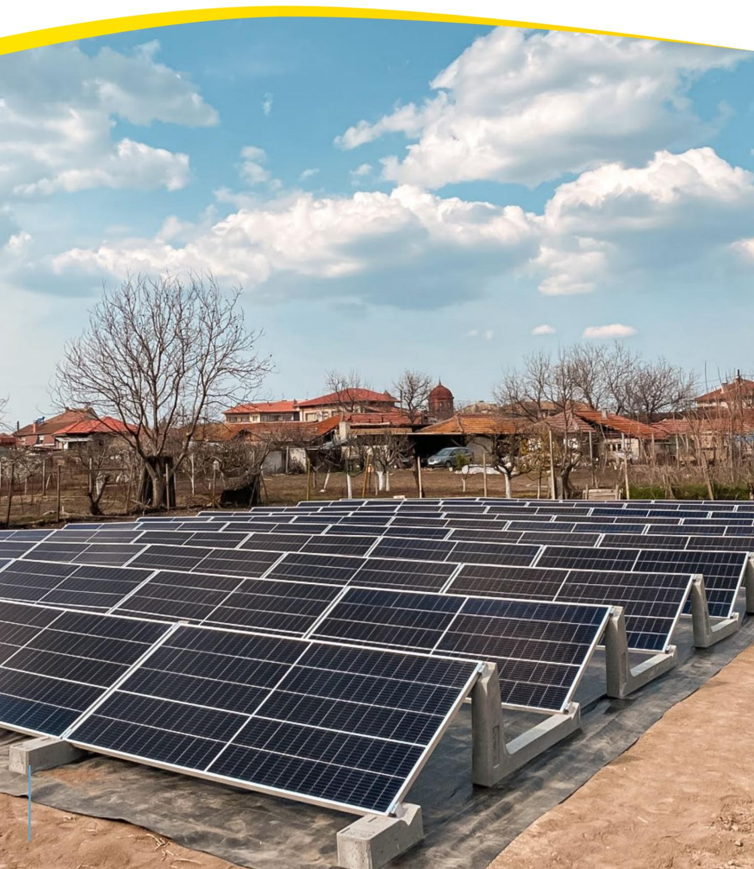
**Basic srl**, is a leading Italian company in the production of structures and accessories for photovoltaic systems. Since 2012 it has offered a valid alternative to traditional systems on the market, presenting an innovative product: Sun Ballast, the support structure for photovoltaic modules on a flat roof.
